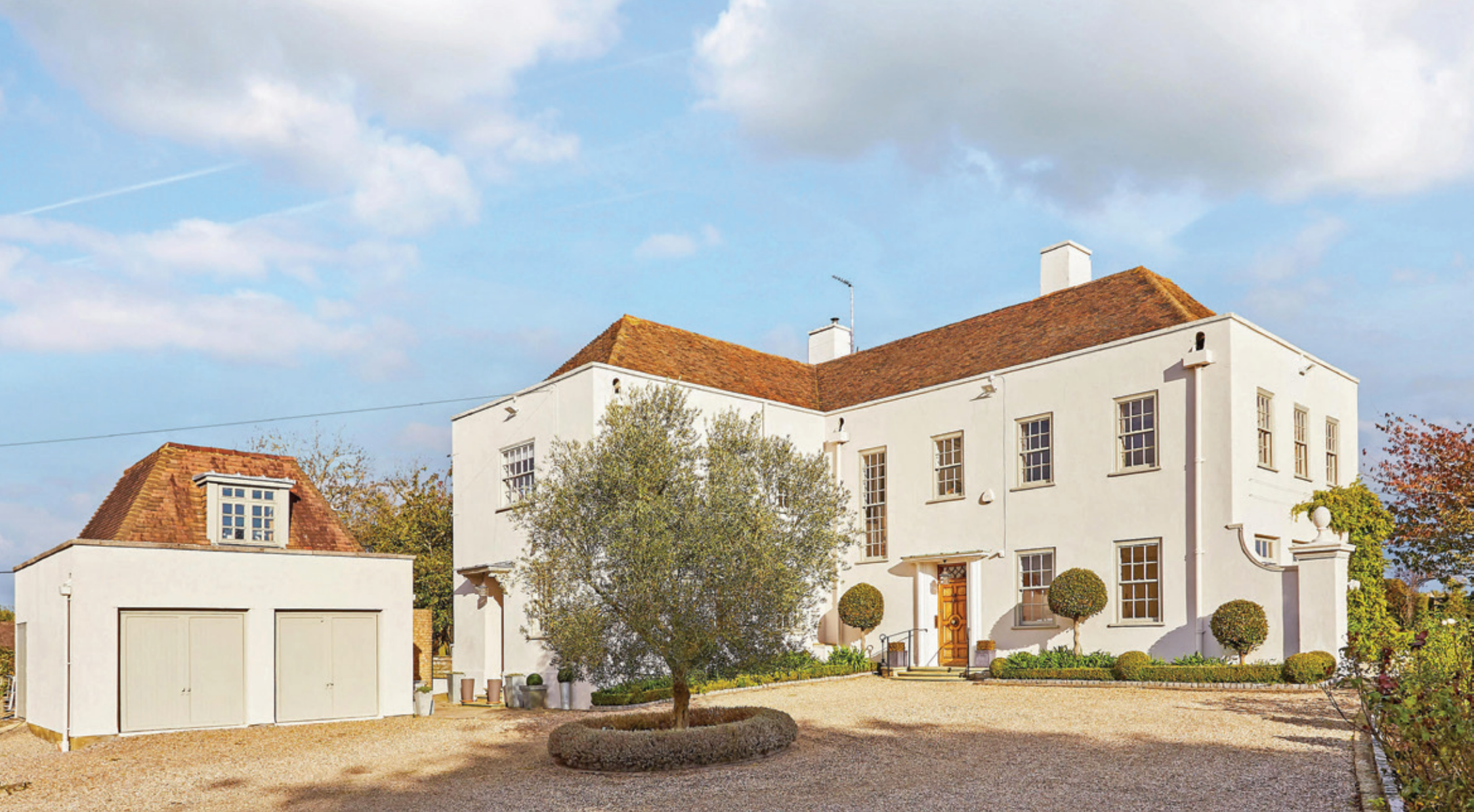
Plumford Farmhouse Plumford Road Ospringe Faversham Kent ME13 0DS
